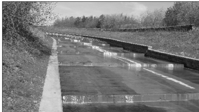
Figure 6. The completed spillway at Ingbirchworth
