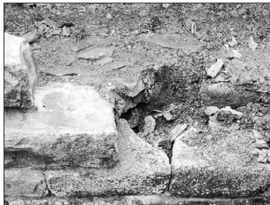
Figure 5. Showing the original wall construction
